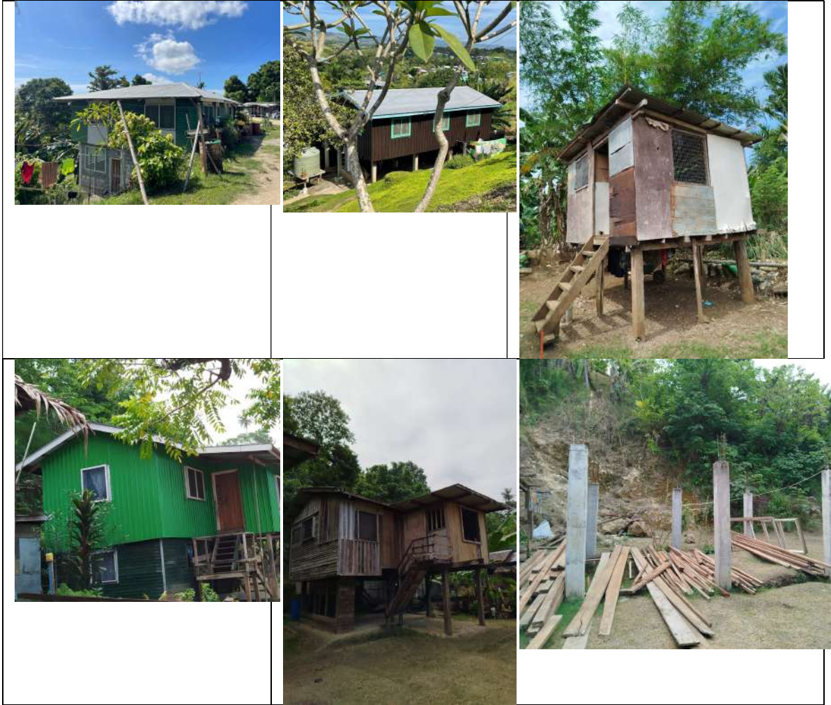
Figure 11.0: Typical Houses inside SIMU property
