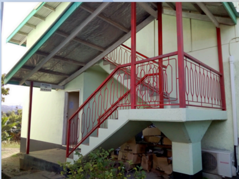
The School of Sciences (SOS) main office building located at the Panatina Campus, East Honiara.
